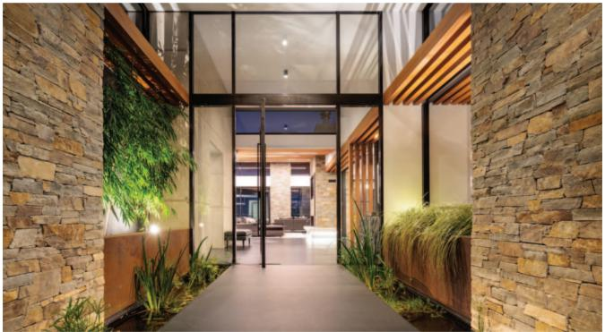
With energy efficient principles at the core, this environmentally sustainable home utilises natural stone and in-situ off-form concrete walling. This methodology was designed to solidify the building whilst using a seamless micro-cement finish on the concrete slab providing the essential internal thermal mass to minimise internal temperature fluctuation.
